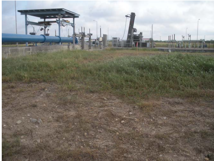
Photo 2: Looking towards Boring B-2
